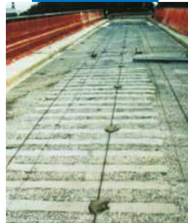
Mapegrout BM-mel fedett Carboplate lemezek
