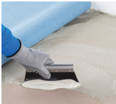
Ultrabond Eco TX1 application
