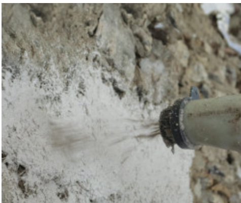
First layer of Planitop Intonaco Armato
