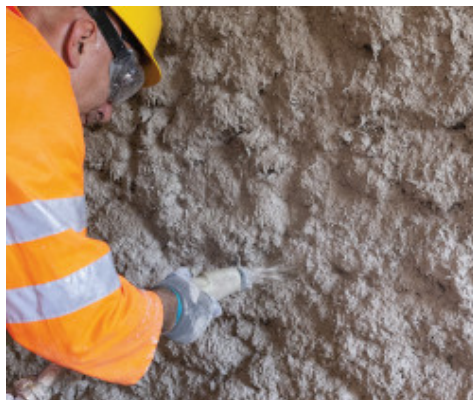
Second layer of Planitop Intonaco Armato
